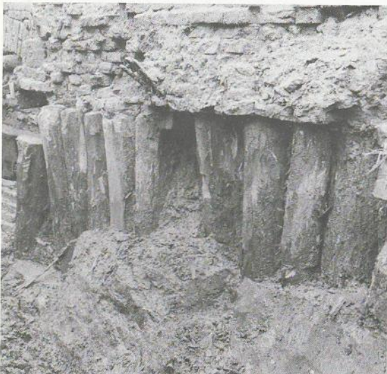
14. detail houten funderingspalen
