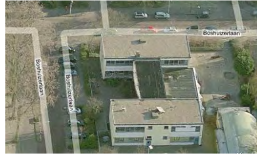
Leiden, Sint Antonius school, Boshuizerlaan 5, 1960 H-school, Arch. Hendriks, Van den Bosch en Hendriks
